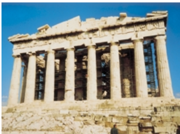
Figure 5.25 Many old and valuable marble statues and buildings in Europe and Asia have suffered the effects of acid rain and have had to be repaired. The Parthenon in Athens, Greece is shown here under reconstruction.
