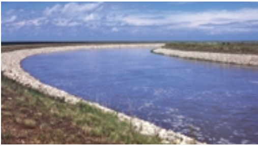
Figure 2.47B Irrigation canals bring water to areas where it is in short supply.
